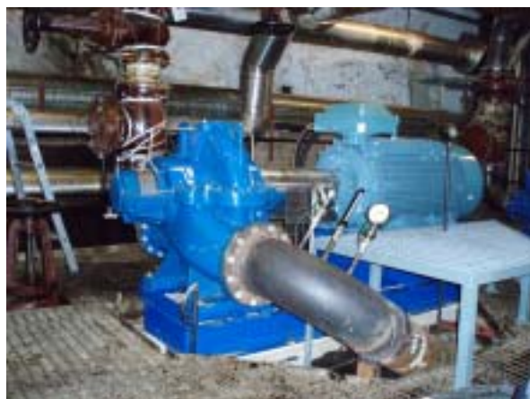
Tjockoljepump Q = 900 \text{ m}^3/\text{h} H = 90 \text{ m}
