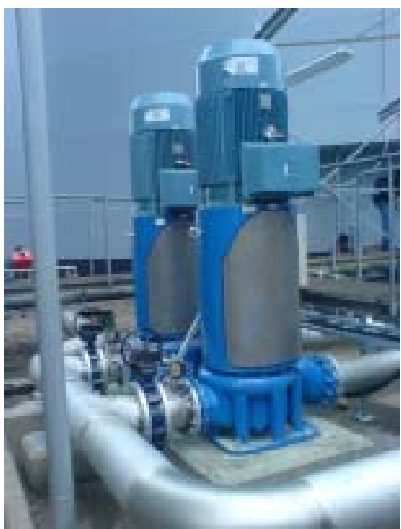
Petroleum pump SNLV-H
